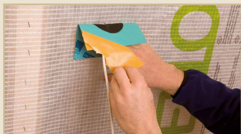
Fig. 90. ROFLEX pipe grommet fixed with TESCON VANA
