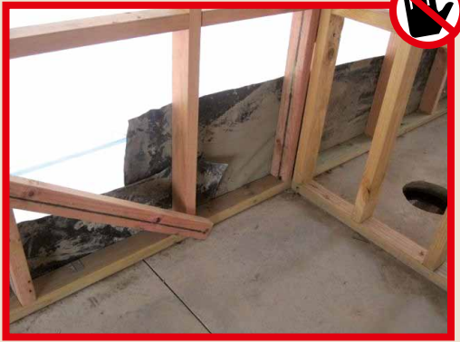
Fig. 79. Bitumen membrane outdoors
