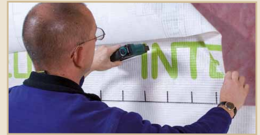
Fig. 86. Taping overlaps
